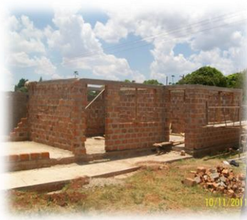
Class block construction continues
