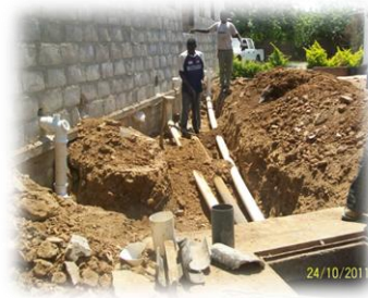
Connecting sewer lines
